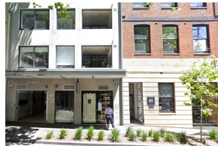
Shopfront of 45 Riley Street and entrance to 41 Riley Street residential
