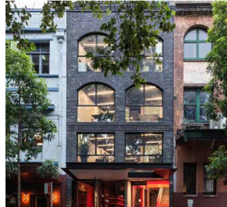
4 storey street wall infill development, 78 Campbell Street Surry Hills
