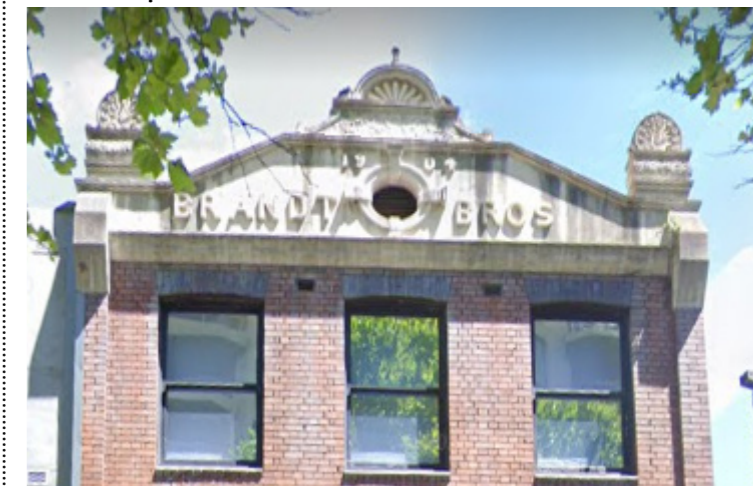
Parapet and upper level windows of 41 Riley Street
