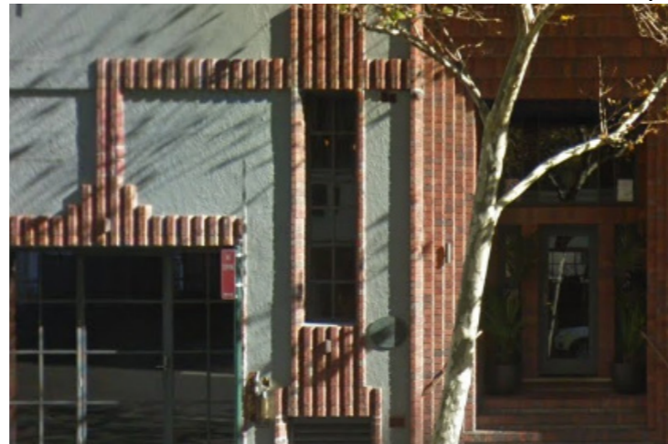
Brick detailing on facade of 55 Riley Street
