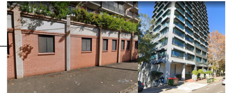
Challenging interfaces with infrastructure
