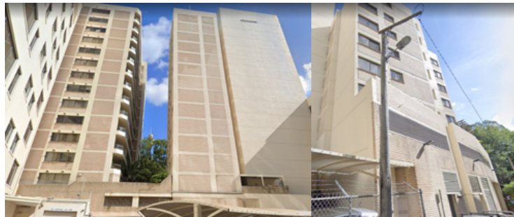
Servicing William Street
