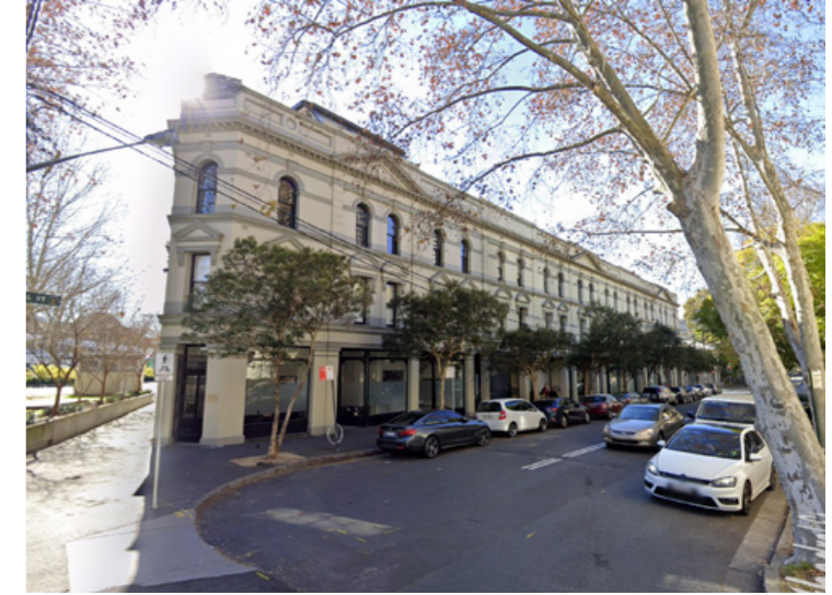
Cathedral Street Character Area, cnr Cathedral and Riley St
